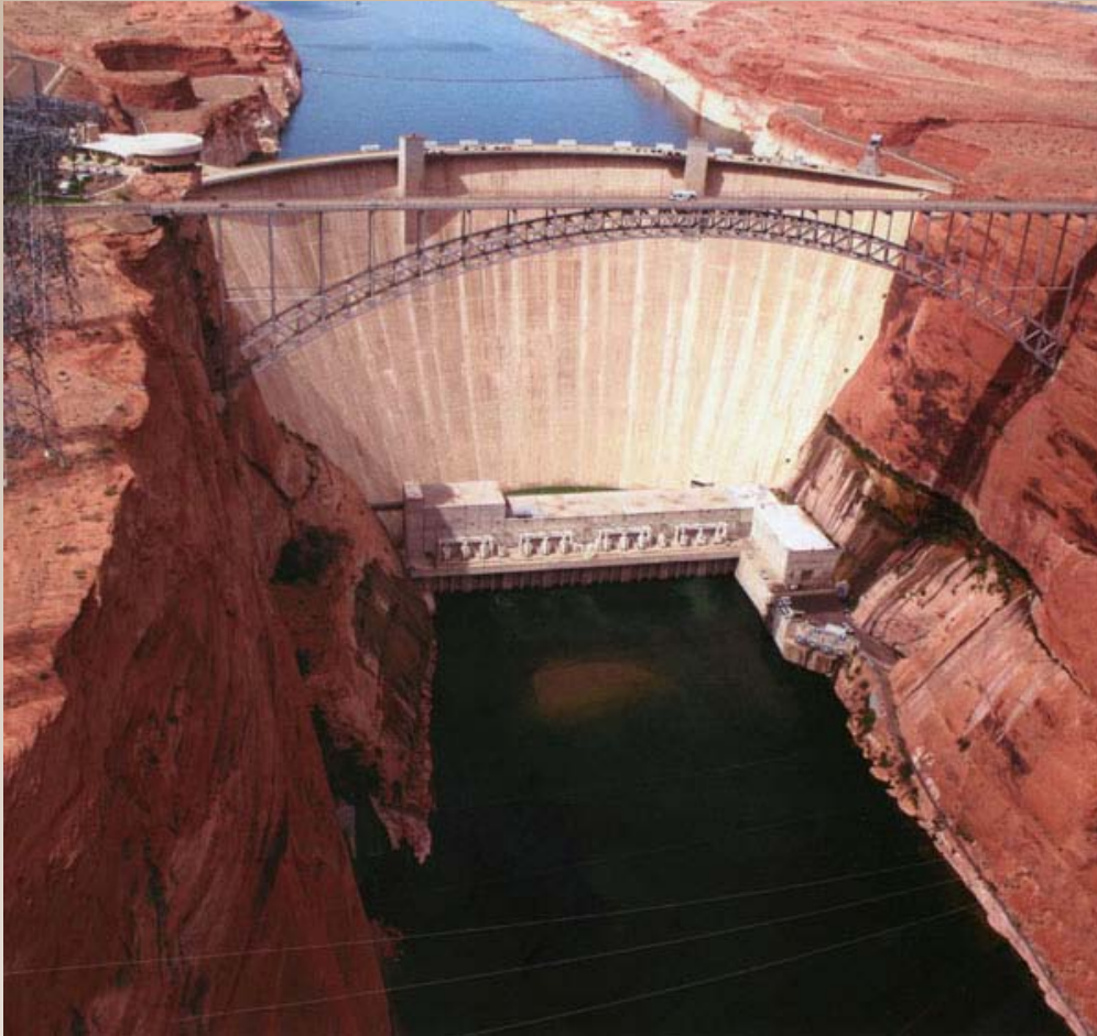
Glen Canyon Dam, Arizona
