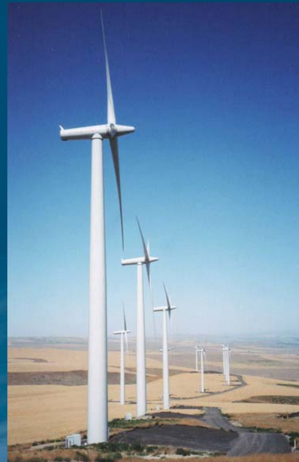
64MW Nine Canyon project, WA Completed December 2005
