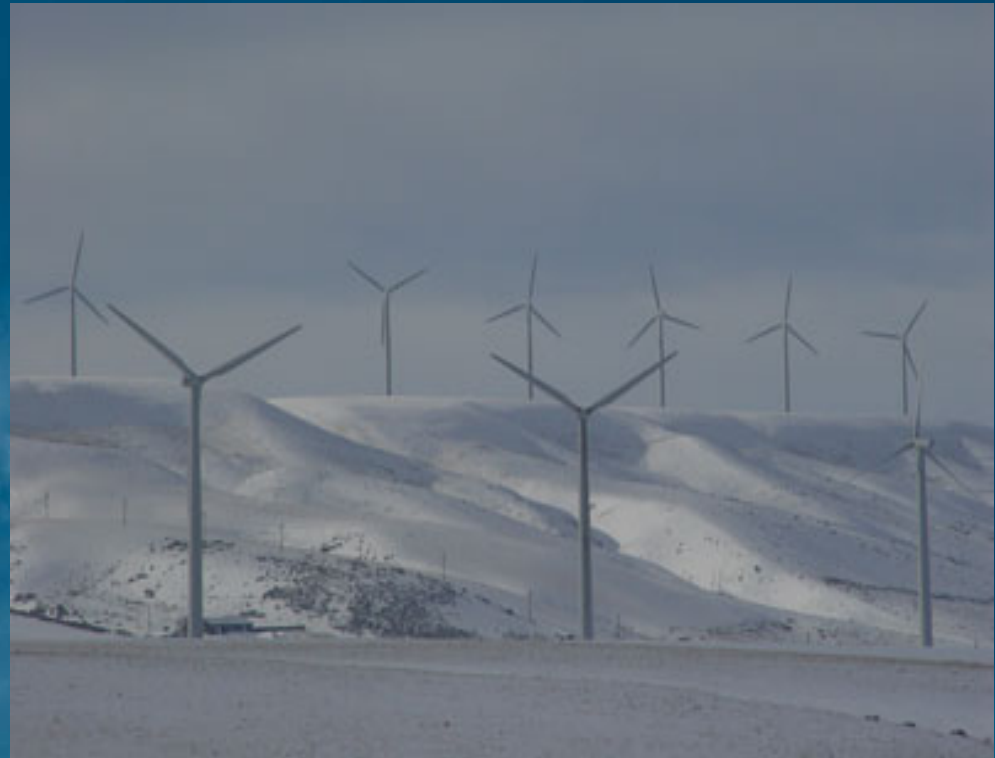
140 MW Marengo I project, WA Completed December 2007
