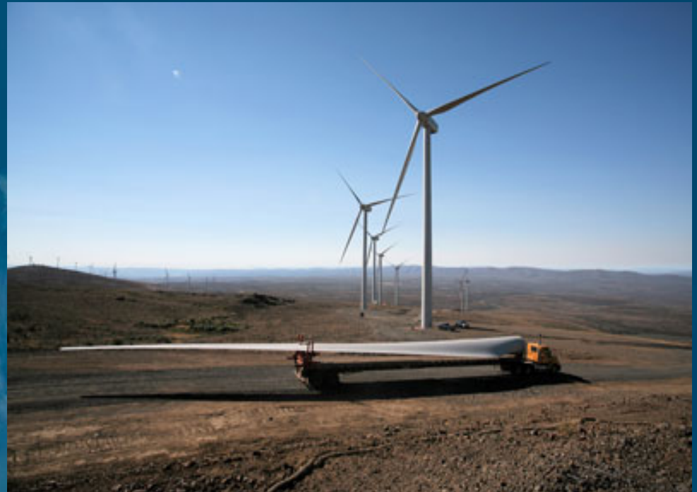
205 MW White Creek Wind Farm Roosevelt, Washington completed 2007
