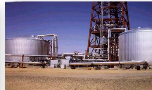
Molten Salt Tanks
